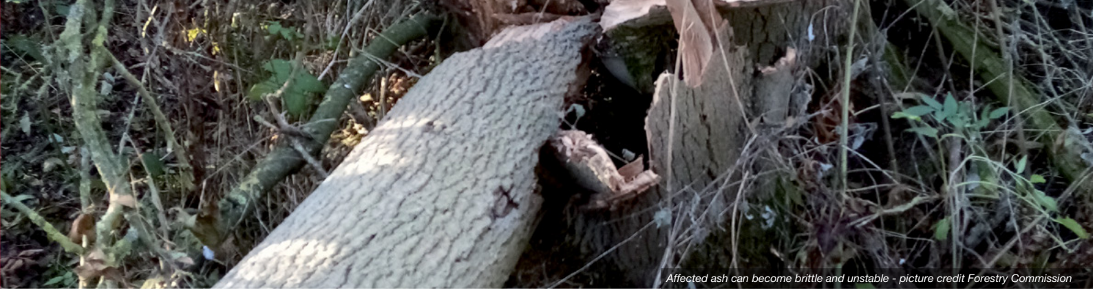
Affected ash can become brittle and unstable - picture credit Forestry Commission
